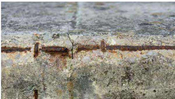
Figure 2: Consequences of reinforcement corrosion
