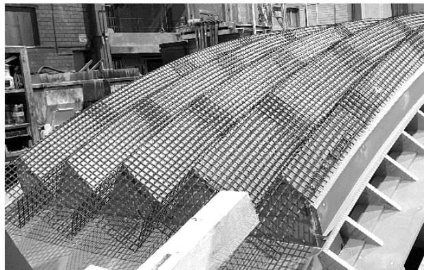
Figure 13: Formed reinforcement grids
