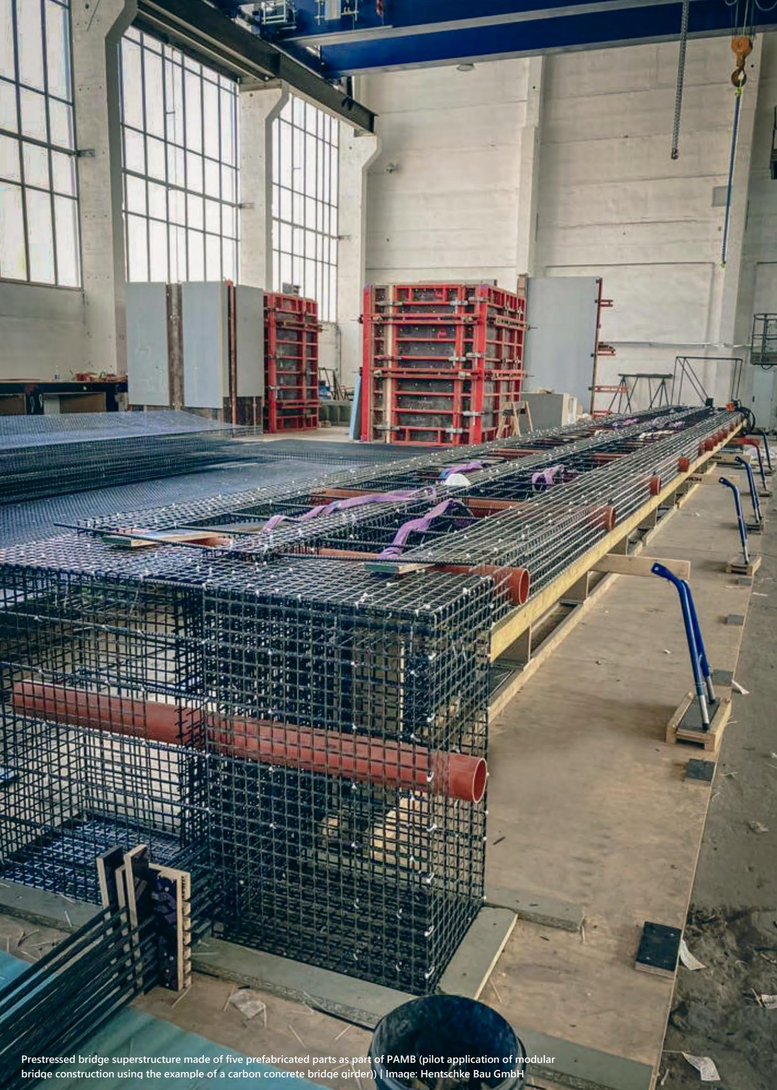
Prestressed bridge superstructure made of five prefabricated parts as part of PAMB (pilot application of modular bridge construction using the example of a carbon concrete bridge girder) | Image: Hentschke Bau GmbH
