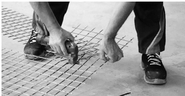
Figure 11: Simple cutting with plate shears
