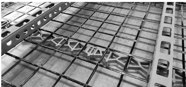
Figure 15: Reinforcement grid with plastic spacers and base made of fiber-reinforced concrete
