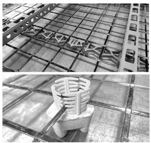
*Figure 15: Reinforcement grid with plastic spacers and base made of fiber-reinforced concrete*
