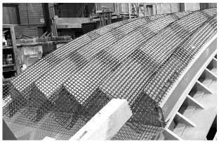
Figure 13: Formed reinforcement grids
