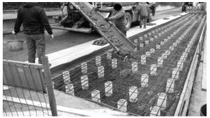
*Figure 14: Plastic filter tubes as supports for a metal-free component*
