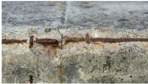
Figure 2: Consequences of reinforcement corrosion
