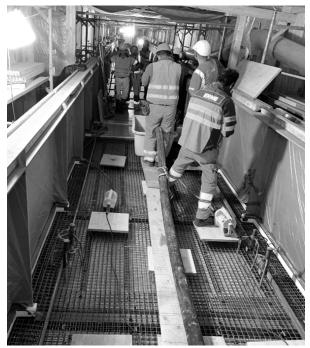
*Figure 19: Access aids to prevent direct access to reinforcement made of fiber-reinforced composites*
