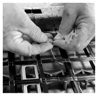
Figure 17: Binding reinforcements with cable ties
